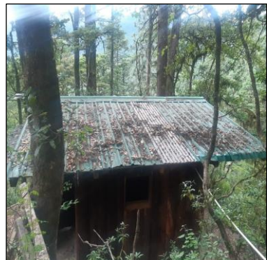
Figure: Restroom two
