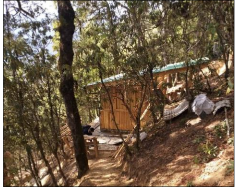
Figure: Restroom two
